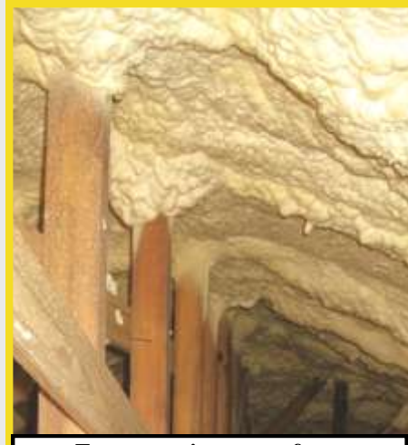
Energy saving spray foam
